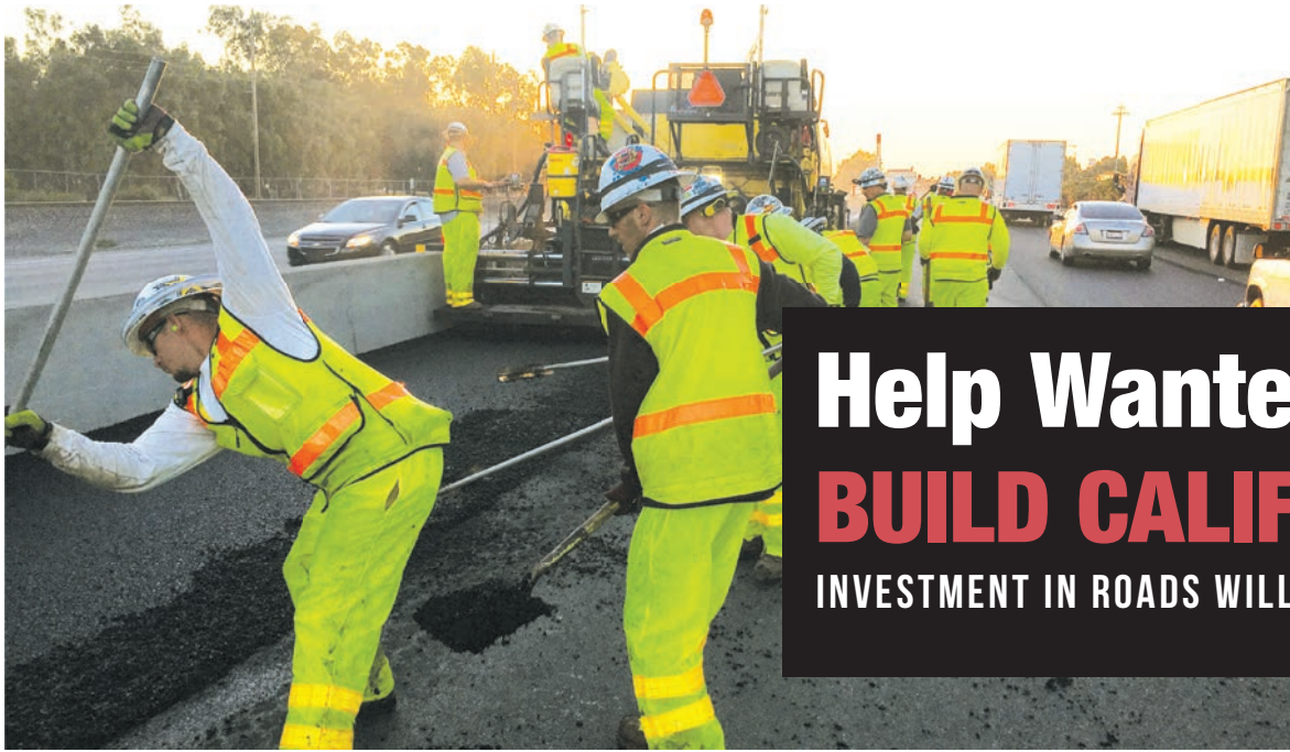
Sacramento residents can expect to see more road construction, like this road resurfacing, as SB 1 funds are put to use on needed transportation projects. PHOTO COURTESY TEICHERT
